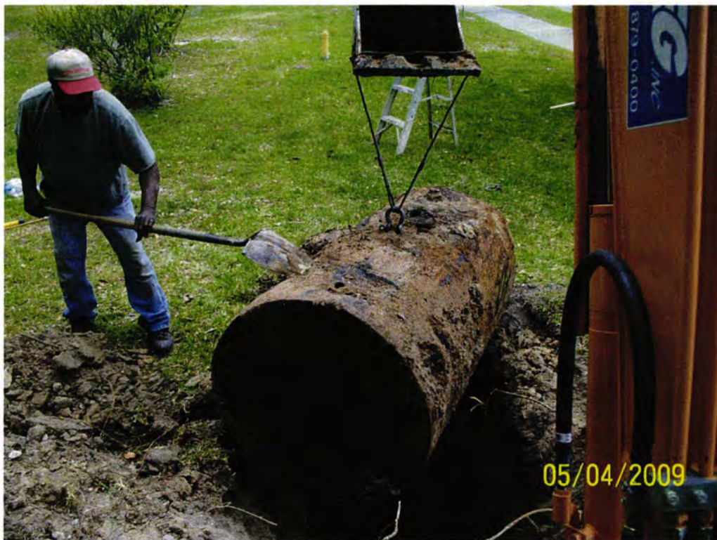
Picture 2: UST 399Acorn-1 being removed from excavation.
